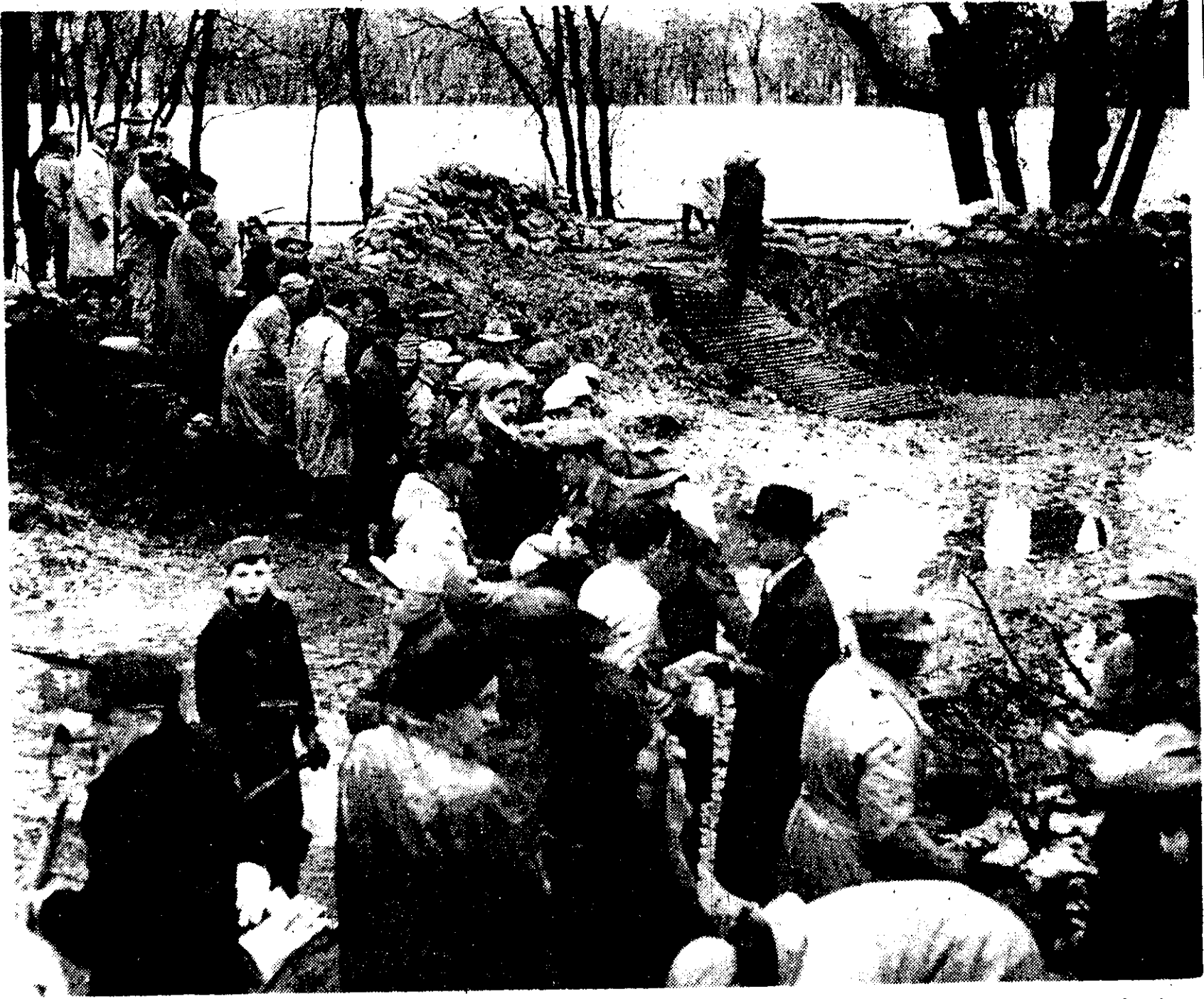
A sudden break-through on the dike at the foot of Helmsdale avenue in East Kildonan occurred about 8 a.m. Tuesday when only half a dozen workers were on the scene. A desperate
