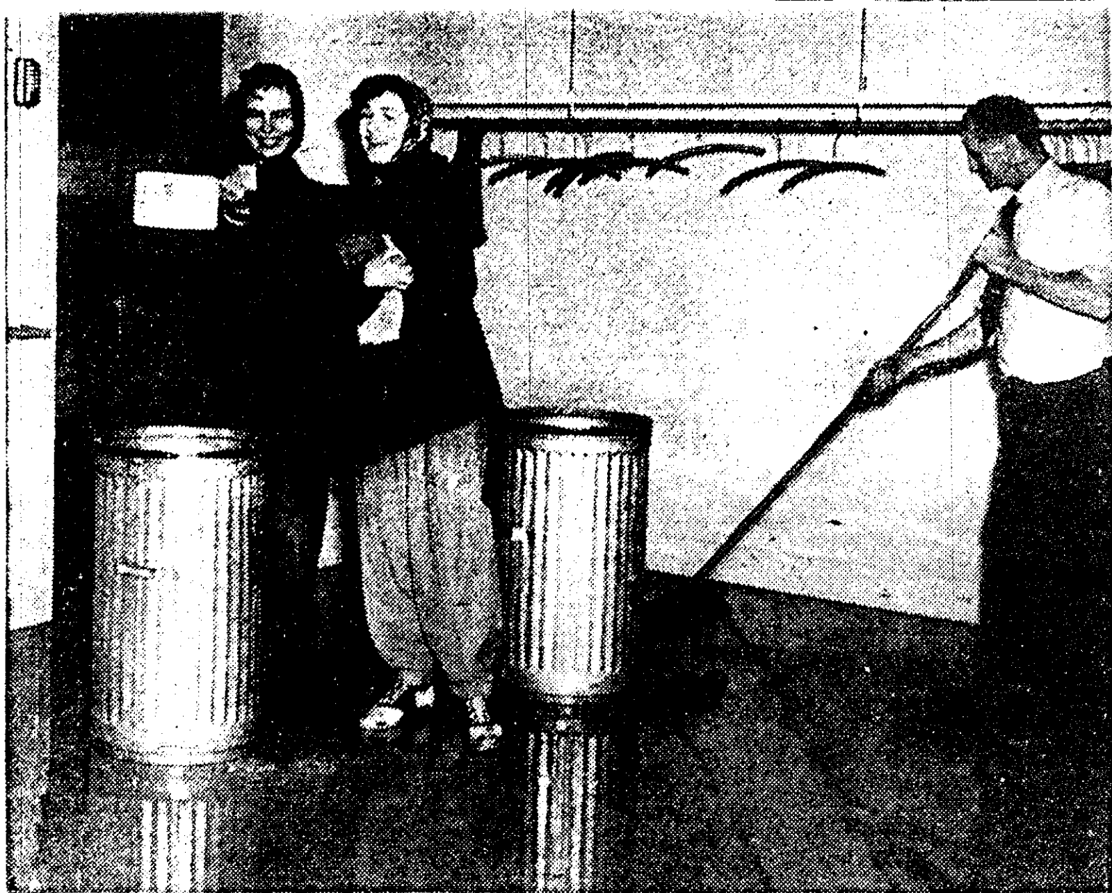
Volunteer cleaner-uppers Doreen Havlick, 16, (left) and Vera Ash, 17, are helping J. S. Thompson, janitor, of Miles Macdonell collegiate in East Kildonan. Paper and asphalt composition waterproof covering was peeled from the centre roof portion of the eight-room, one-storey structure by the high winds Monday. While workmen repaired the damage, 25 student volunteers with brooms pushed Tuesday's rain down hallways into washroom drains, while the main student body, numbering 200, took an unexpected holiday. School is expected to resume again Friday.
