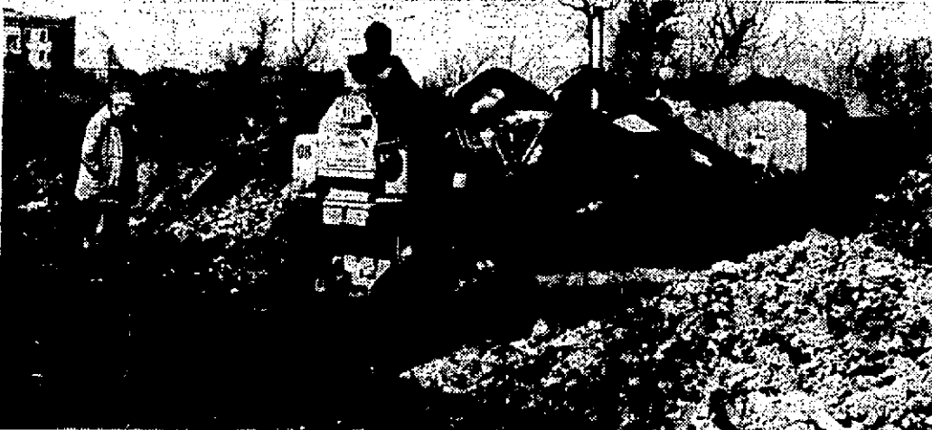
Bulldozer operators Frank Frampton (standing) and Alphonse Corriveau of city engineer's department building dike along Red river bank, near Arnold avenue, Fort Rouge.
