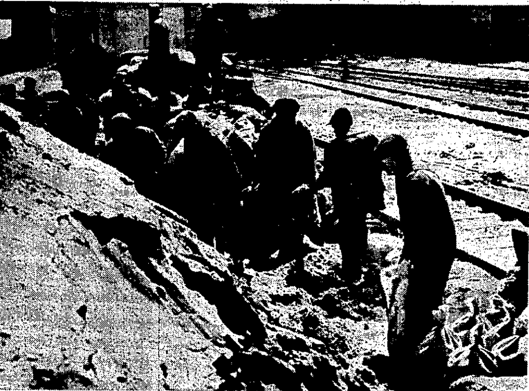
Crew at city yards, Tecumseh street and Ross avenue, loading sandbags for flood walls.
