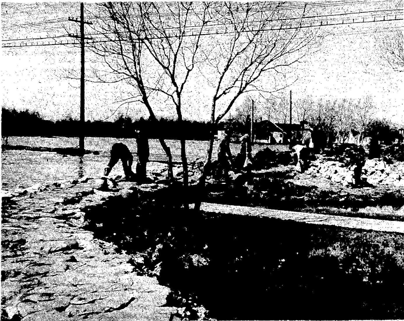
Rough winds buffeting the flood water against this thin line of sandbags at the Fort Garry dike, crossing the Pembina highway was termed "extremely hazardous" Thursday by army engineers. Feverish activity to build the weak section higher can be seen as men pile bag after bag against the crushing wall of water.
