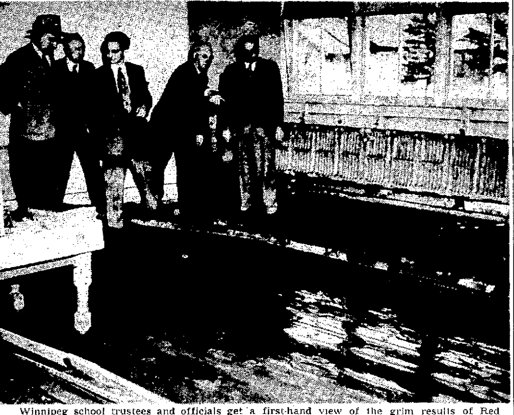
Winnipeg school trustees and officials get a first-hand view of the grim results of Red river flooding in the old annex of the Riverview school during an inspection trip. A buckled section is noticeable in the centre-foreground. Taking in the scene (left to right) are: W. A. Martin, commissioner of buildings; F. A. Alden, secretary-treasurer; J. Zuken, school trustee; G. P. Macleod and P. C. Jessiman, school trustee and chairman of the building committee. The inspection was made Monday.
