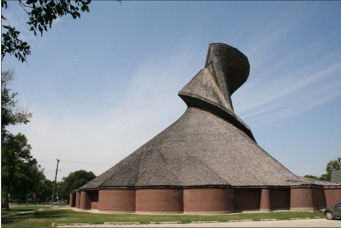
Plate 26 – Precious Blood Church, 200 Kenny Street. Built in 1967, it is undoubtedly one of Gaboury’s finest and most recognized designs, 2012. (M. Peterson, 2012.)
